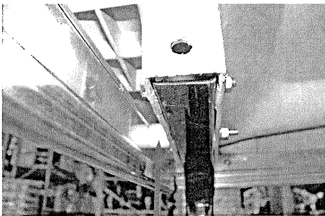
1/2" Spacer Placement
